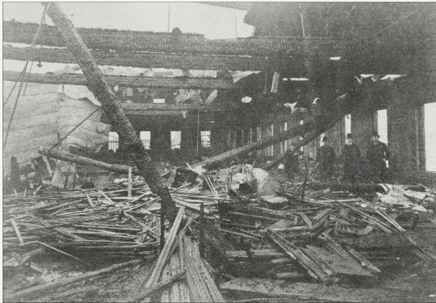
On March 2, 1854, the boiler that fed the machinery at the Fales & Gray Car Works in Hartford exploded, killing 16 workers and injuring many more. Connecticut Historical Society, Hartford, Connecticut
