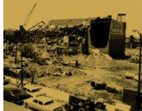
State Theater being demolished, 1962. Hartford History Center, Hartford Public Library
