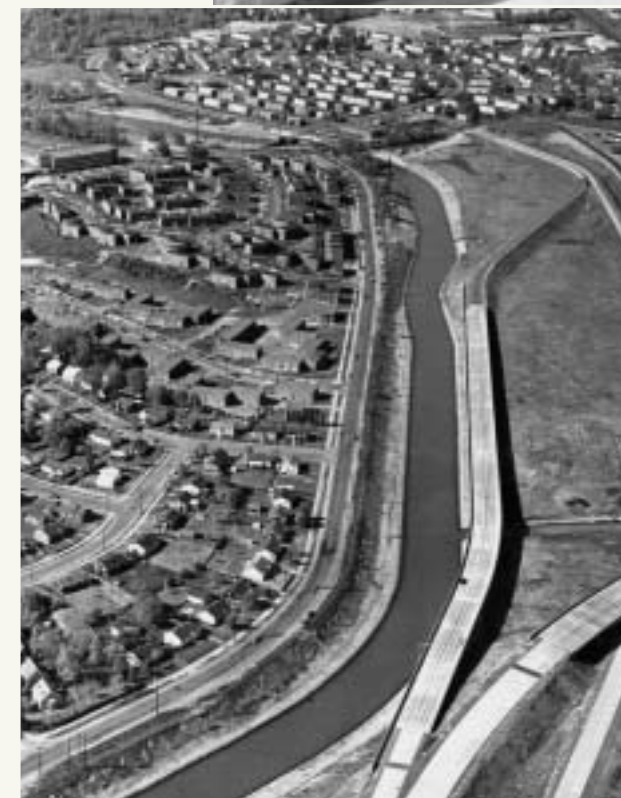
top pf page: The Park River becomes a river of concrete after being buried underground in twin concrete conduits. The 1833 stone arch bridge still carries Main Street over the conduit; Hartford Public Library would be built over this spot in 1957.
